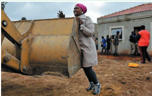
A woman tries to stop a bulldozer from demolishing her house in Lenasia. Picture courtesy of Associated Press
